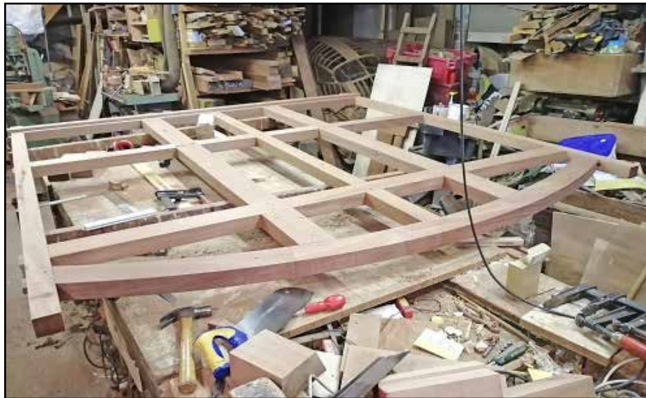
All the framing has been machined and trial fitted at Andrew Daniel's Harrogate workshop. Here is one of the ends of the Fish Van showing the roof profile. The framing was then dismantled and taken to Pickering for final re-assembly. Photo: Andrew Daniel.
