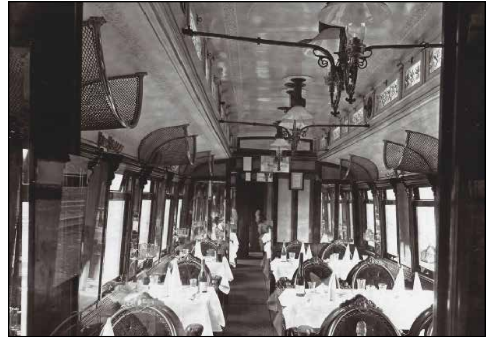
This is what 189 will look like one day. Can you help with the Lincrusta border? If you look on the lower ceilings, you can see, just in front of the curved luggage nets, the Lincrusta border. There are similar ones on either side of the clerestory ceiling, running the full length of the saloon. Can you help us procure a modern equivalent? Photo: LNERCA Collection.
