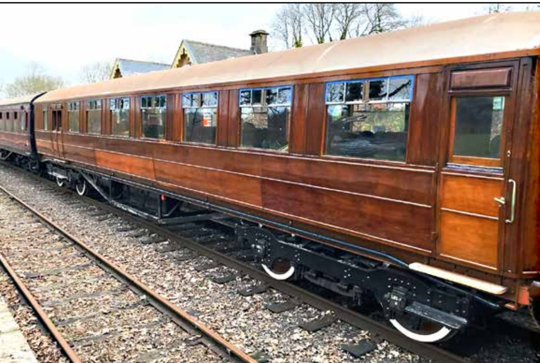
A close-up of 43632 at Wirksworth, Ecclesbourne Valley Railway. The newly installed double doors, to allow wheelchair access, are at the far end of the carriage. There was still much work to be undertaken - and remedied - before it could be said that this Cold War survivor was ready to take passengers once again - over six decades since it had last done so. Photo: Nick Stringer.
